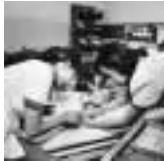
BINTARO INTERNATIONAL HOSPITAL; JAKARTA, INDONESIA
